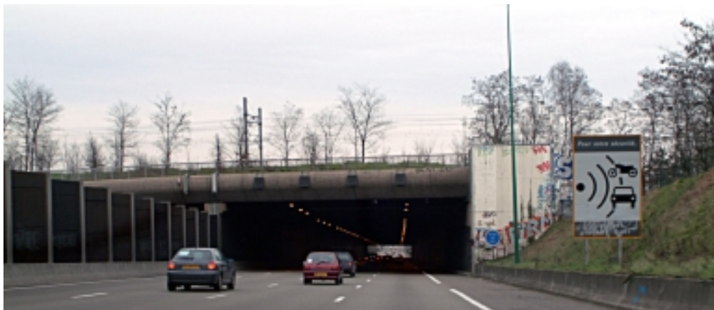
Approach to the cut and cover road tunnel at Versailles – this is the location for both road and terrorist attack synthesised incidents involving fire
