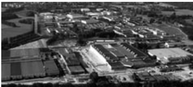
Figure 7.3 - Urenco's Almelo centrifuge enrichment plant has no associated power plants or cooling towers. 170
