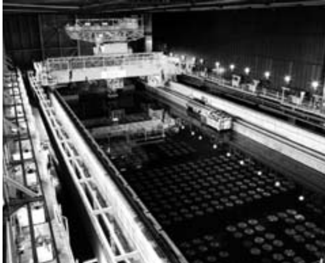
Figure 5.2. Spent-fuel storage pool at the U.K. Thermal Oxide Reprocessing Plant (THORP). [Source: World Nuclear Association.] 163
